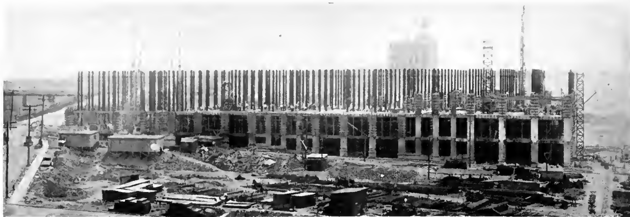
PROGRESS VIEW Showing erection of steel columns
